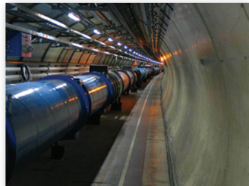
Accelerator Magnets in the LHC Tunnel
