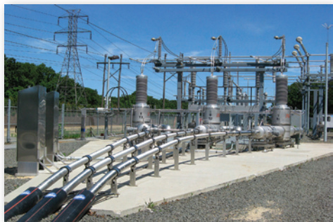
138kV HTS cable system installed in Long Island, NY Image courtesy of American Superconductor
